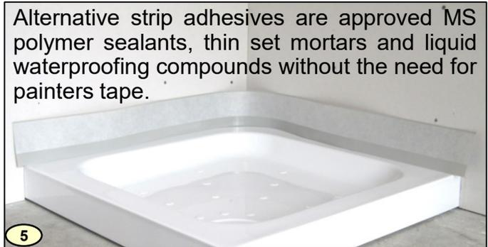
**4.** Draw wall lines through wall marks. These two lines define the adhesive bed upper and lower boundaries. **5.** Measure and cut the strip to extend between the receptor end lines.
