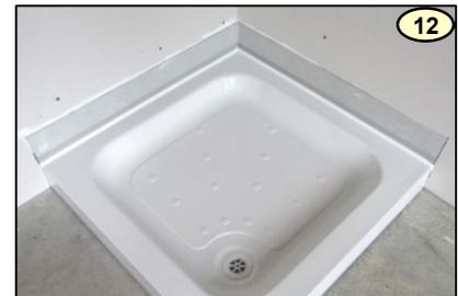
**9-10.** Apply Sealux-N (or equivalent) over the first side strip/rim junction and rub up the silicone to form a 9/32" (7mm) fillet over the joint. Repeat this joint sealing process on each remaining side.
