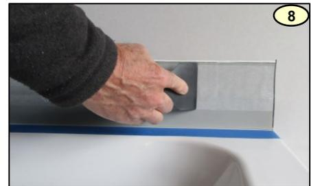
**6-8.** Apply a zigzag line of an approved adhesive sealant between the wall lines and spread using the serrated edge of the spatula to form an adhesive bed. With the strip resting on the rim, progressively touch-engage the strip with the adhesive bed. Use the spatula straight edge to firstly press the strip into corners and then firmly against each wall to form a permanent bond. Remove the painters tape off the wall if applied.
