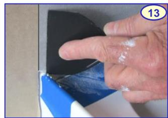
If using a non-silicone sealant, thin set mortar or liquid waterproofing compound as the strip adhesive, do not mix that adhesive with the silicone applied into the joint. In 1 and 2-wall enclosures, the process of bonding the strip to the wall and joint silicone (10-13) should be done diligently before the silicone has skinned. In 3-wall enclosures, this process can be done in stages.
