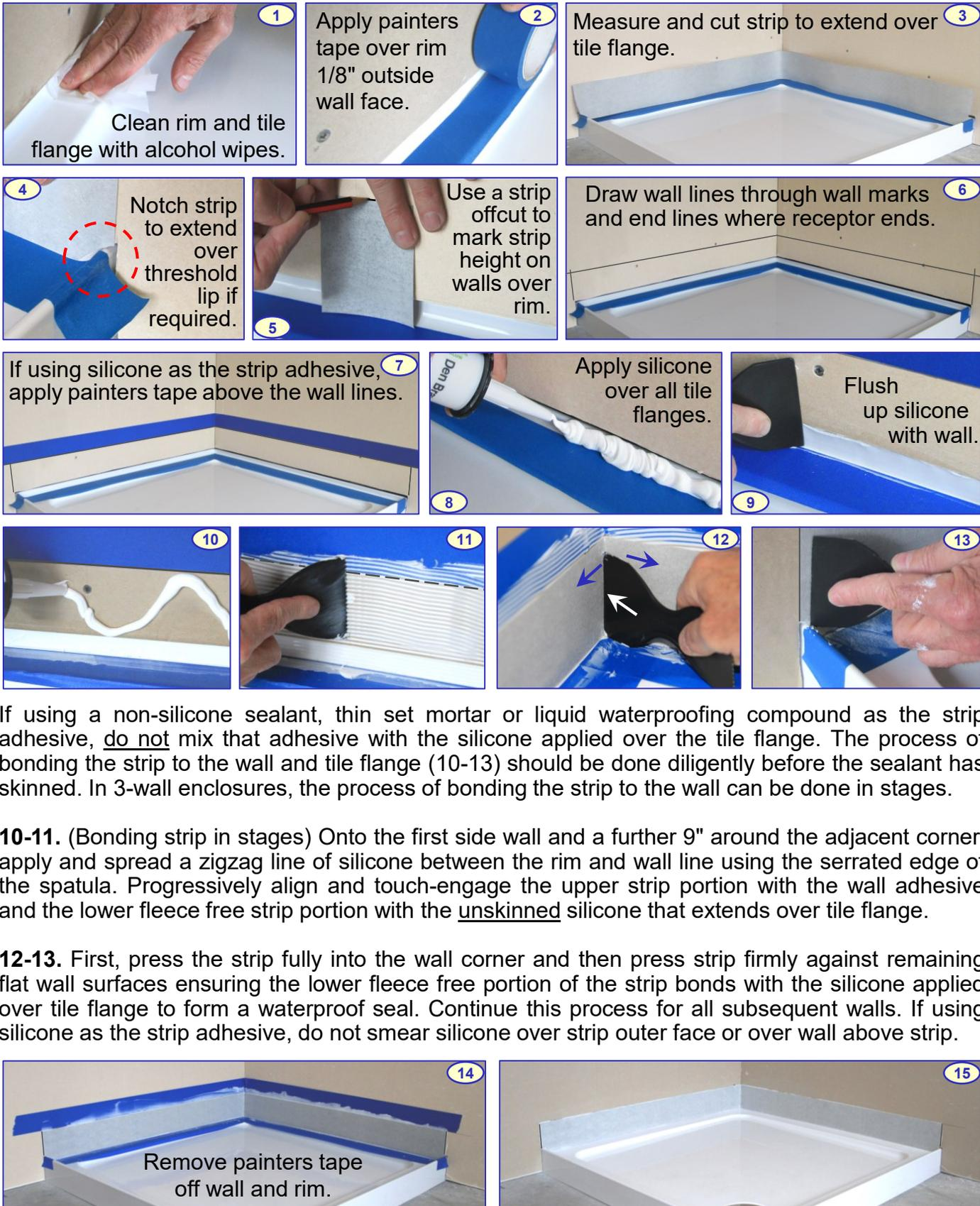
If using a non-silicone sealant, thin set mortar or liquid waterproofing compound as the strip adhesive, do not mix that adhesive with the silicone applied over the tile flange. The process of bonding the strip to the wall and tile flange (10-13) should be done diligently before the sealant has skinned. In 3-wall enclosures, the process of bonding the strip to the wall can be done in stages.
